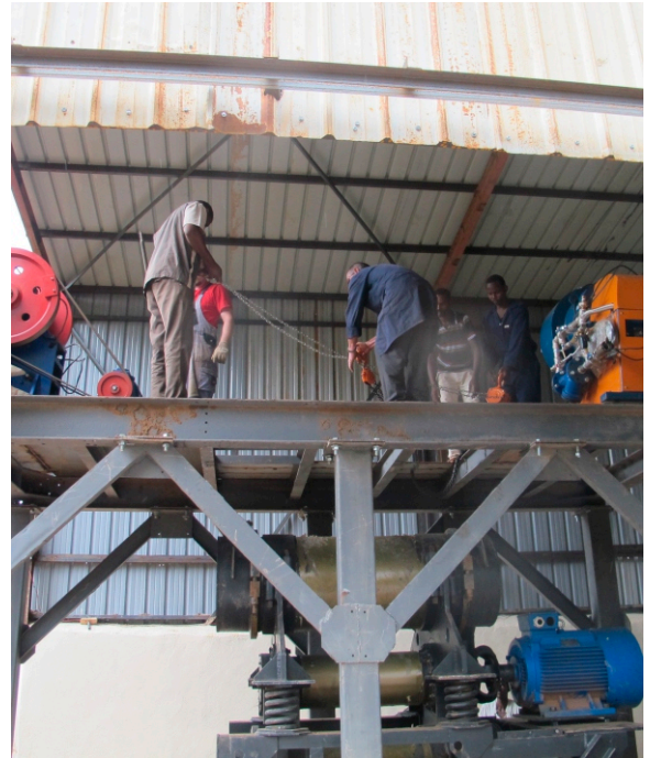
Sudan, installation processing complex
