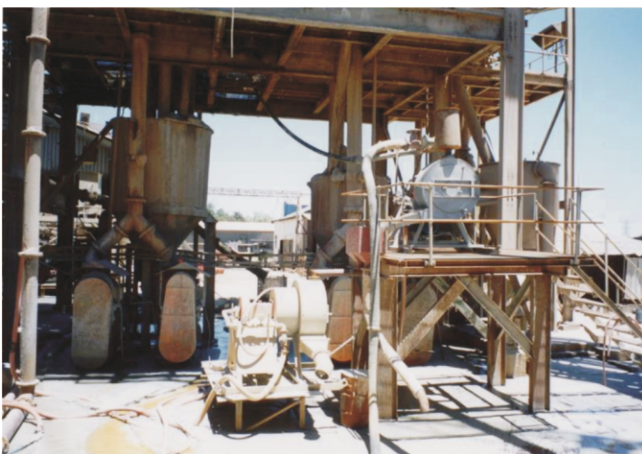
"ITOMAK-KN-1,0" in operation
