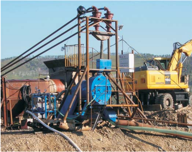
Installation for fine gold recovery from tailings, Zabaykalye
