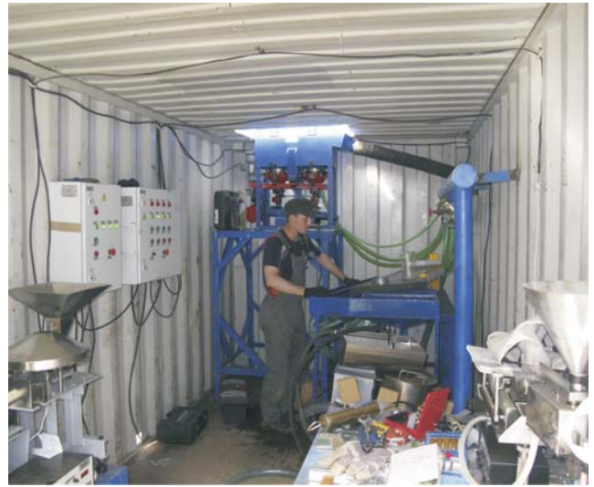
Installation for final retreating of gold concentrates
